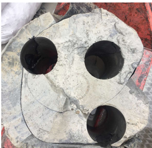
Рис. 3. Места отбора кернов раствора из тела опытных буринъекционных свай Fig. 3. Places where mortar samples were taken from the shaft of experimental drill-injection piles
