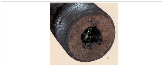
Fig. 1. Tubing with paraffin deposits on the inner surface
