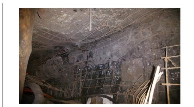
Fig. 7. Failure types of the elements of props and rocks in ventilation drift 2-7
